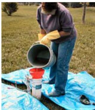
► Pour the mixture into the well and avoid spilling on any wire connections. A funnel should be used for pouring the chlorine solution into small openings.
