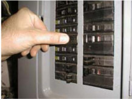
► **Turn off electrical power to the pump by turning off the circuit breaker or unscrewing the fuse.** If the breaker or fuse box has a “lockout” hasp to prevent someone from accidentally turning on the water pump circuit breaker, use it. **Power should not be turned back on until STEP 6 or after the chlorine solution has been placed in the well.**
