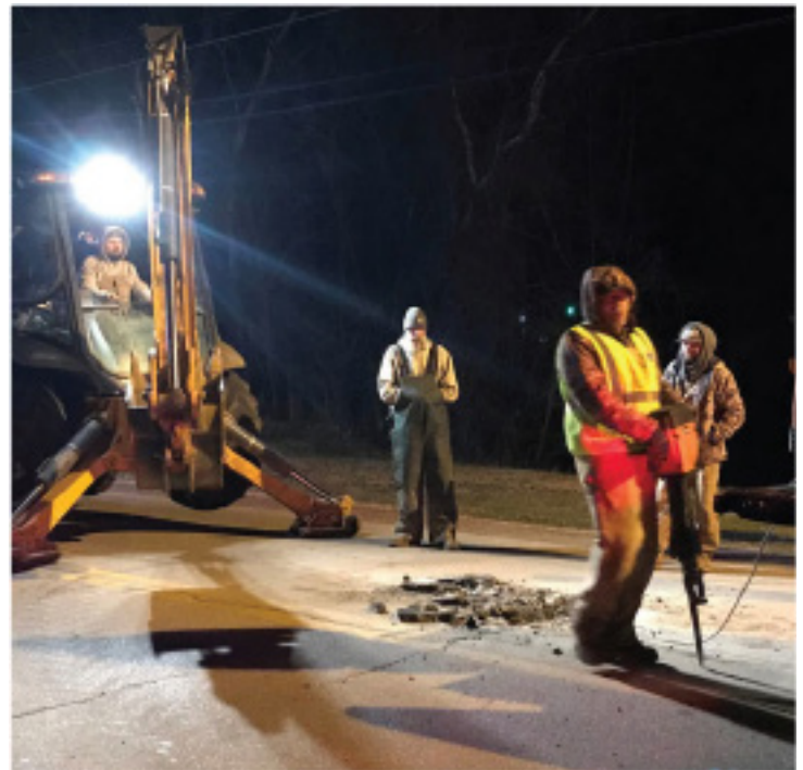
Joe takes a turn with the jackhammer during an emergency.
