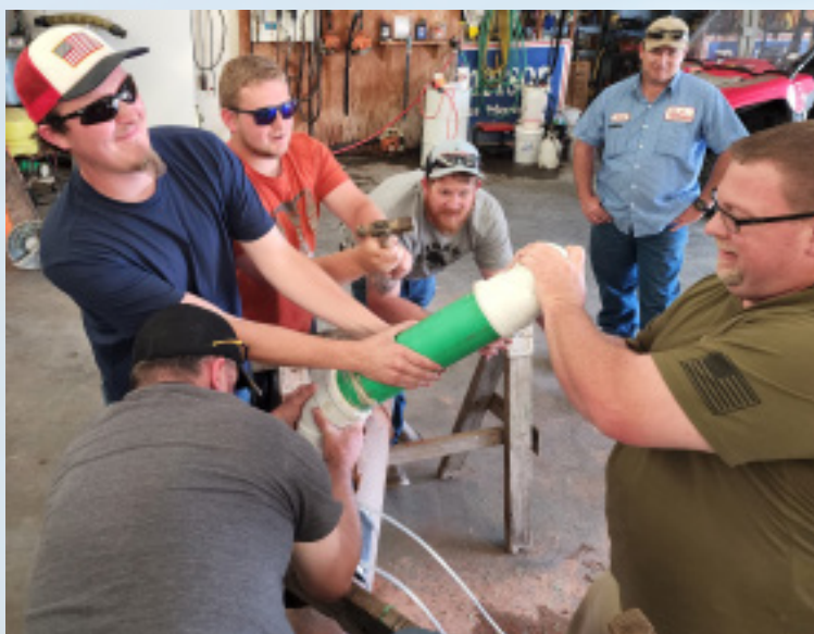
Delta Regional Authority Wastewater Apprentices receive Hands-On wastewater tap training.
