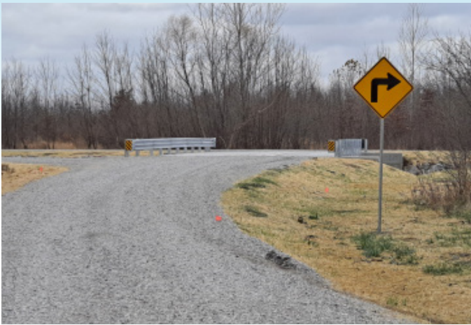
Replacement Hauns Mill AOP Bridge
